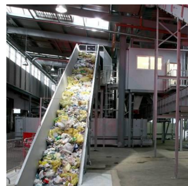
Photo: Waste sorting plant
