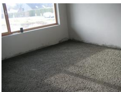
Photo: Bound EPS ballasting
